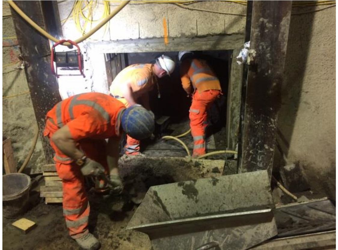
Timber Headings underneath Kennington Loop Complete in Park and green SCL section
