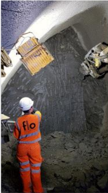
SCL Pilot tunnel Complete
