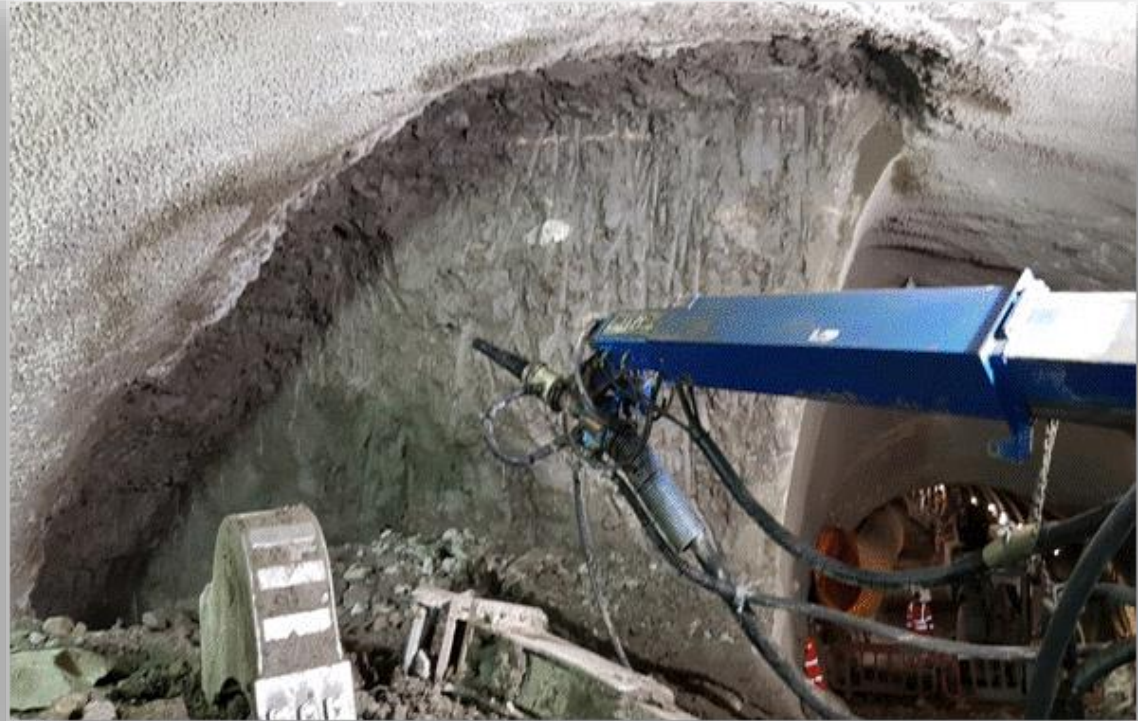
Spray concrete lining (SCL) Complete
