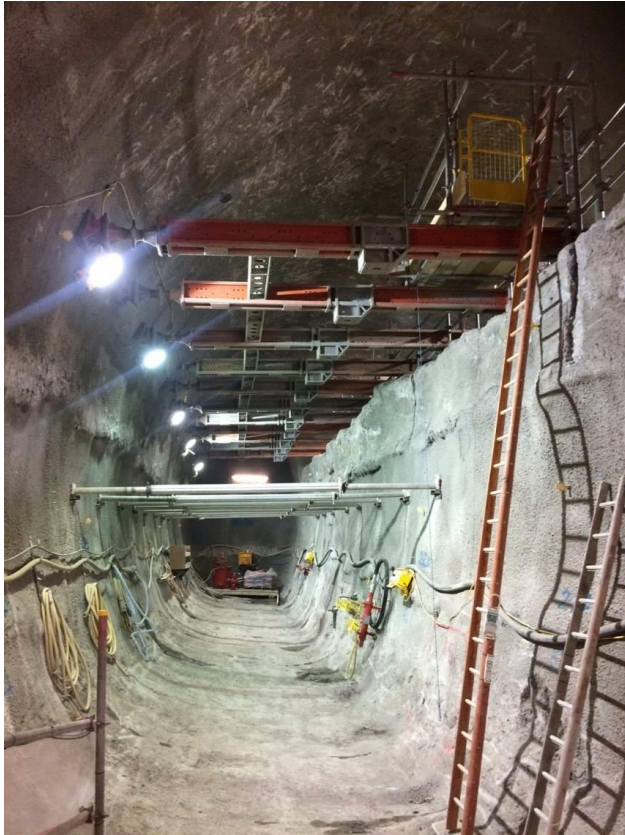
Sprayed Concrete Lining SCL Completed in Park and Green
